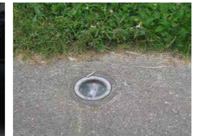
Solar studs integrated in the ground
